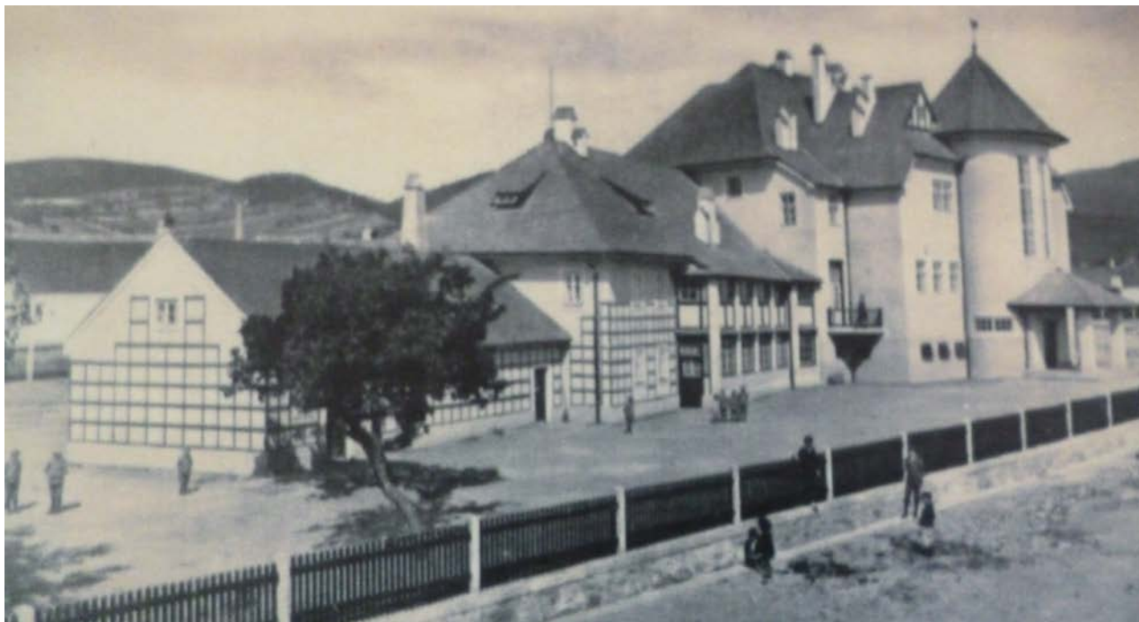
Figure 1: Historic photograph of the orphanage, in front: ancient living part of the mill (source: Petronela Pagáčová).
